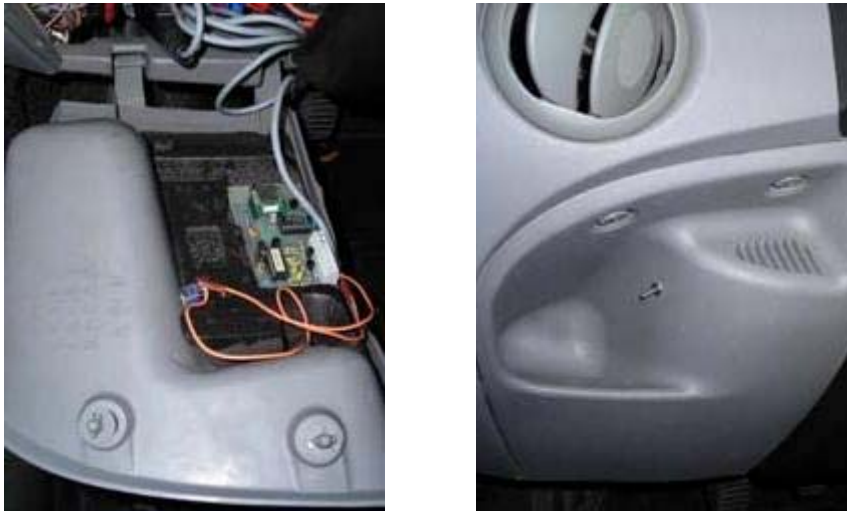
Fig. 1. Our scan tool has been fixed to the door of the fuse box (left). The power switch is accessible from the driver's seat (right).
